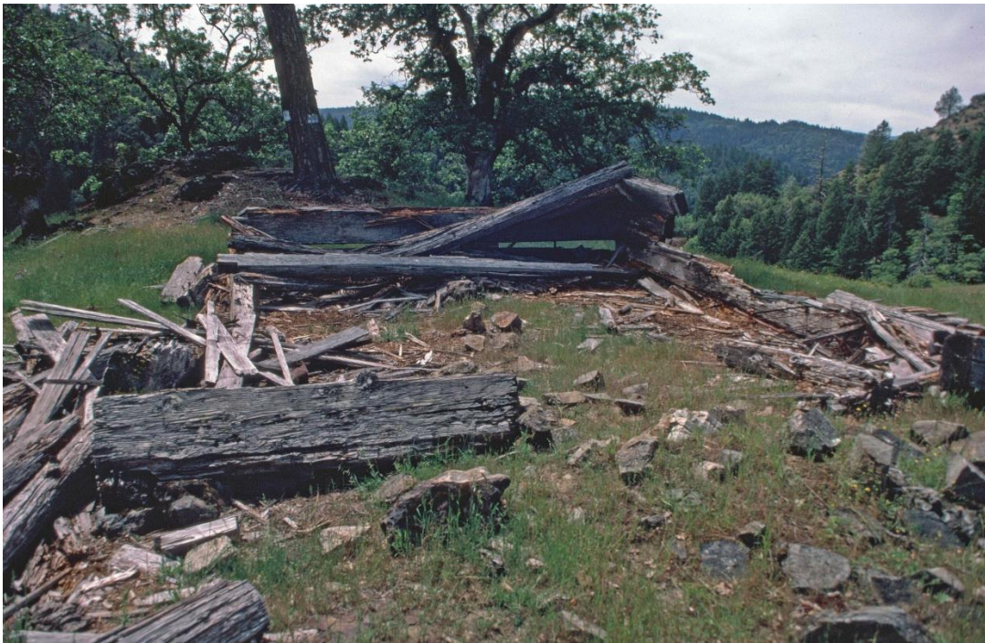
View to northwest of cabin remains. (T. Keter May 1986)
