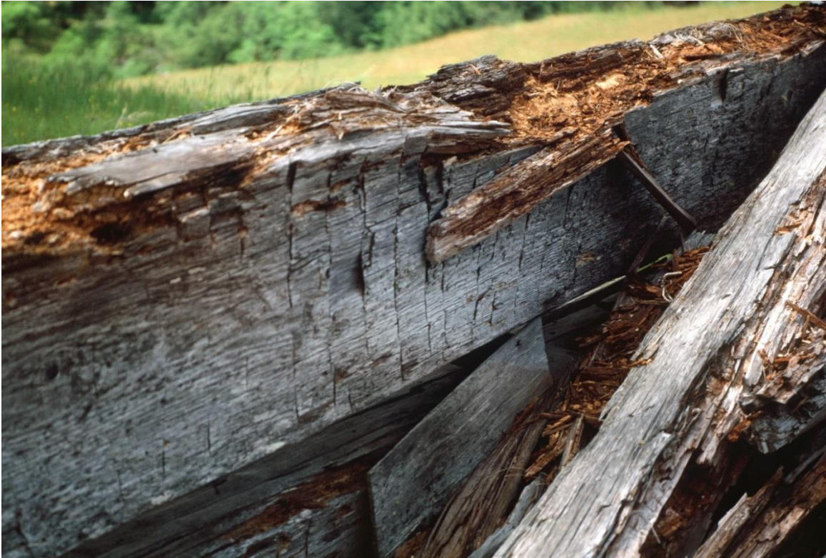
View to northwest of cabin remains. (T. Keter May 1986)
