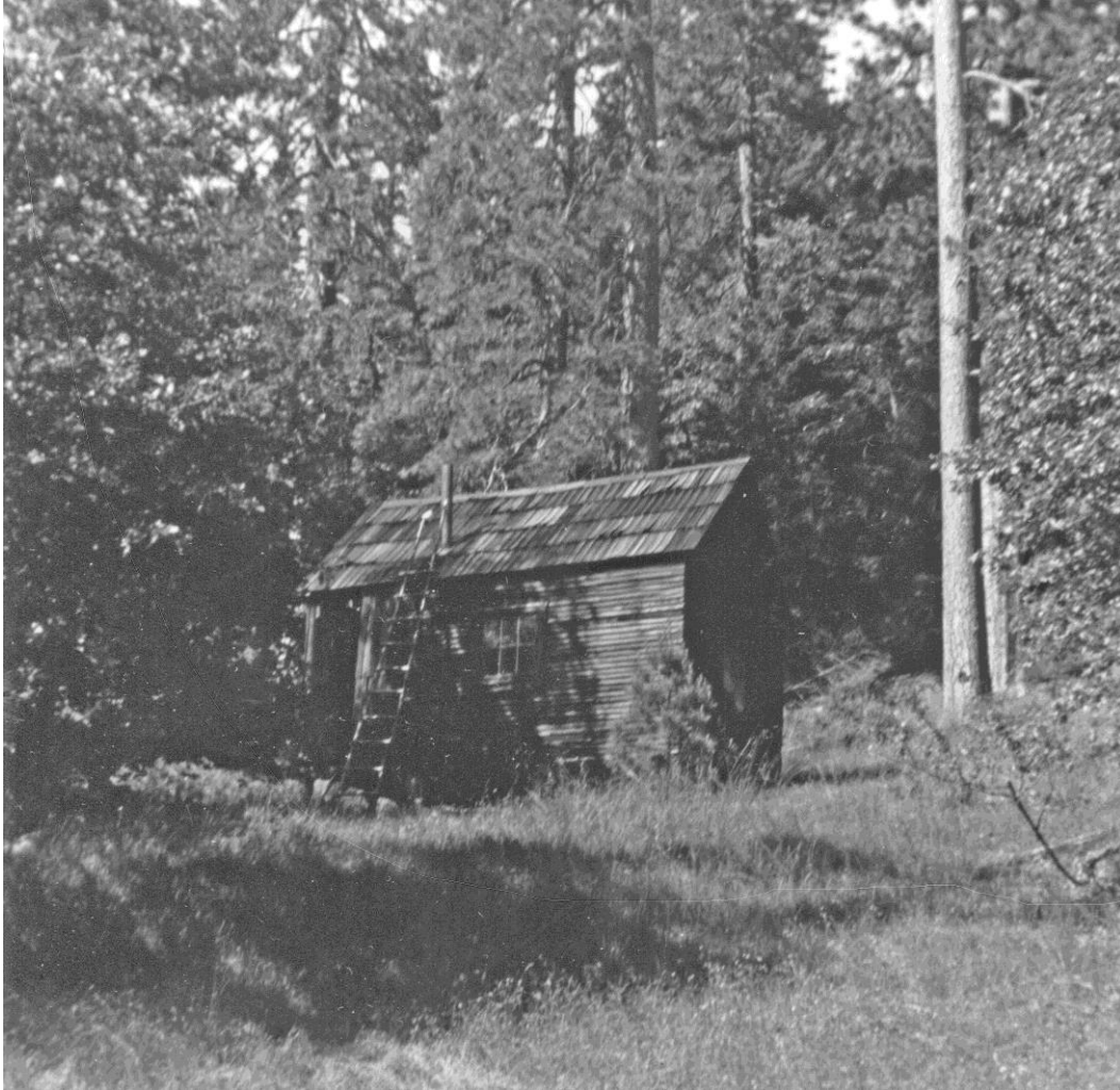
Image 4-10 Dan East Cabin c1940 (Stapp Photograph Collection)
